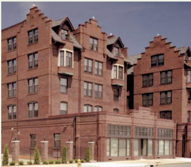
New Holland Apartments, supportive housing in Danville, developed by Crosspoint Human Services
