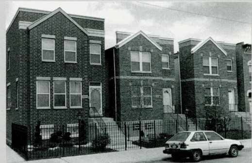
Brand-new townhomes in the West Haven community.
