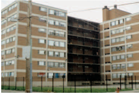
Pre-Redevelopment: Ogden Courts
