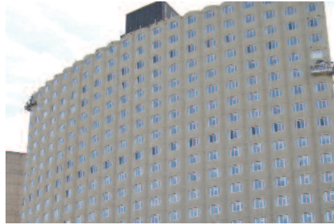
Post-Rehabilitation: Hilliard Towers Apartments
