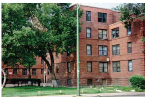
Pre-Redevelopment: Lathrop Homes
