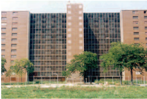
Pre-Redevelopment: Rockwell Gardens
